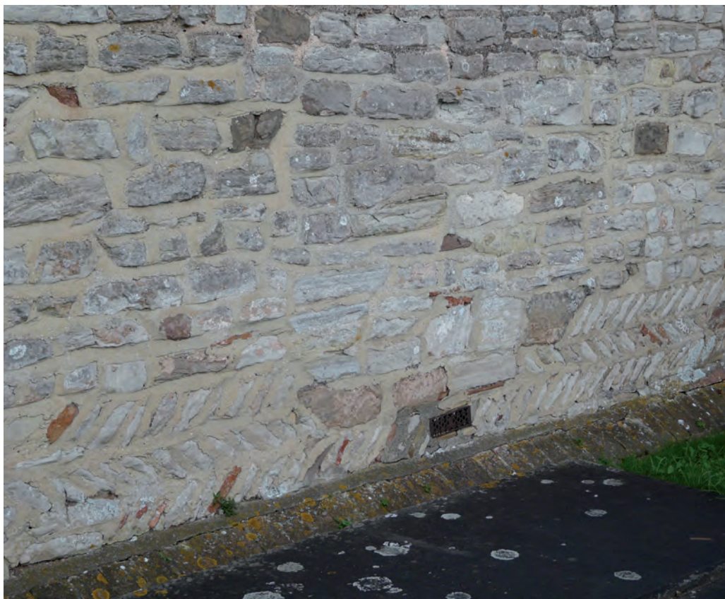
Fig. 2 South wall of the nave of the church of St James, Staunton
