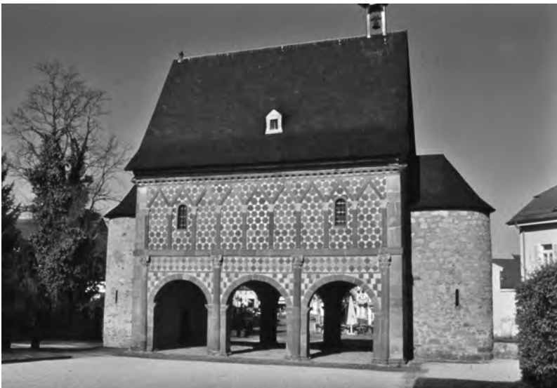
Plate 5: Mid 9th-century gatehouse in forecourt of abbey of Lorsch (Hessen, Germany).
