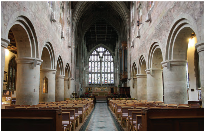
Fig. 10 Great Malvern Priory, looking east, showing in the foreground the retained Romanesque arcade in the nave, and the re-worked, Perpendicular choir beyond. Copyright Bob Embleton and licensed for reuse under the Creative Commons Licence
