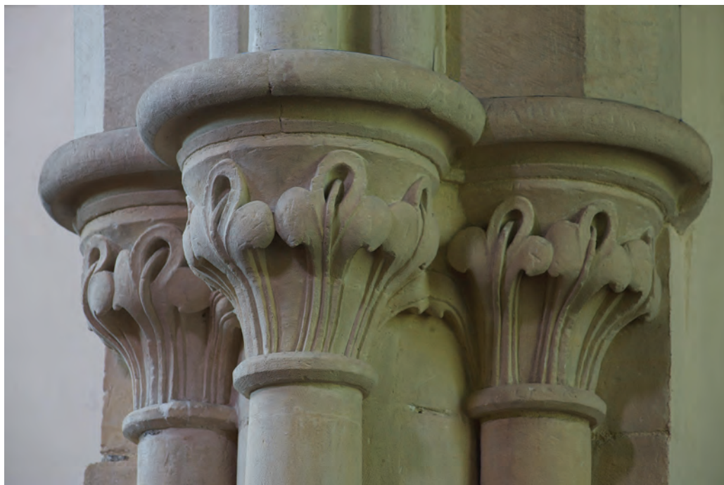
Pl. 40 Deerhurst, St Mary's Priory Church, N nave arcade, pier N2, E capitals
