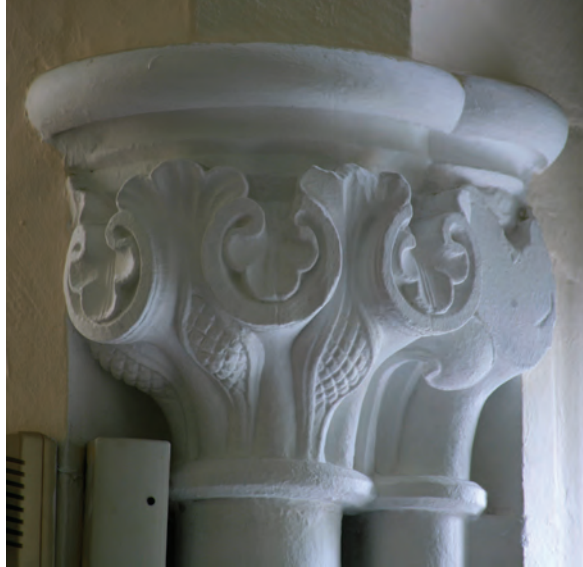
Pl. 41 Gloucester, St Peter's Abbey (now cathedral), Abbot's Lodging (Church House), W hall, first floor, S capital of S window
