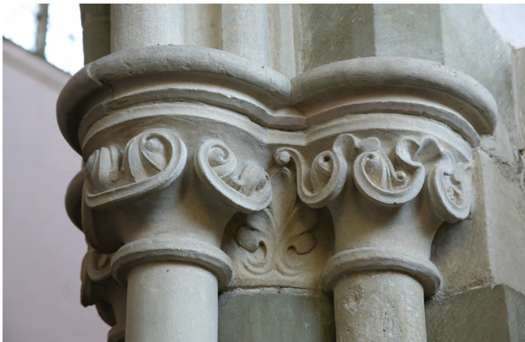
Pl. 32 Deerhurst, St Mary's Priory Church, S nave arcade, pier S2, detail W capitals from SW
