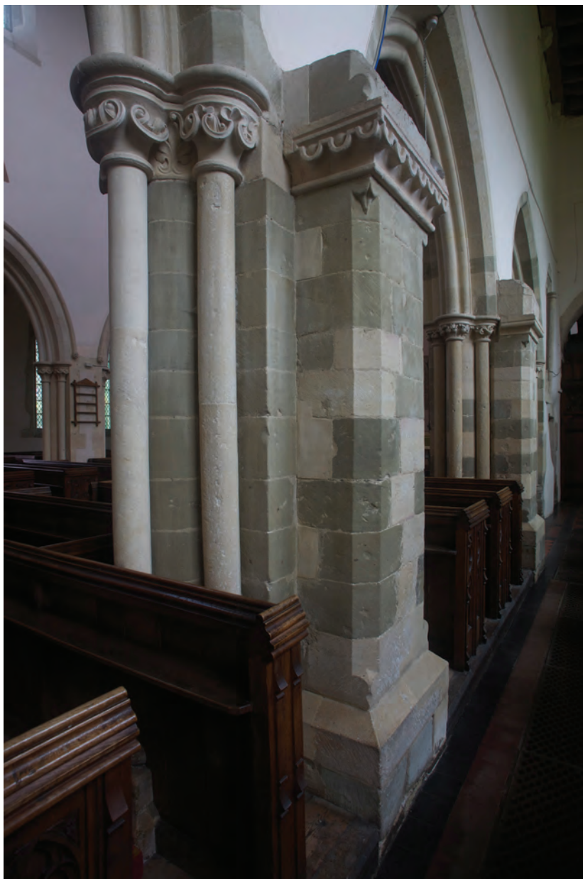
Pl. 28 Deerhurst, St Mary's Priory Church, S nave arcade, pier S2 from SW
