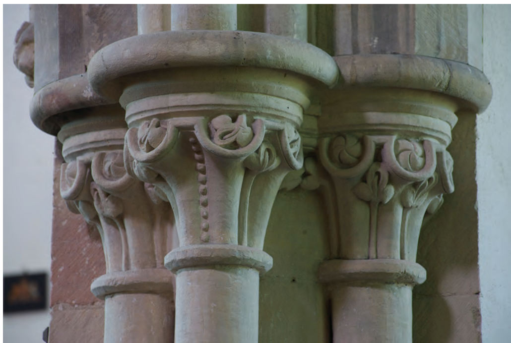
Pl. 39 Deerhurst, St Mary's Priory Church, N nave arcade, pier N1, E capitals
